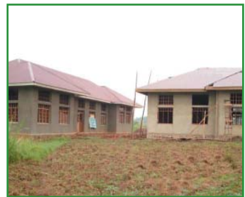
New operating theatre & intensive care
